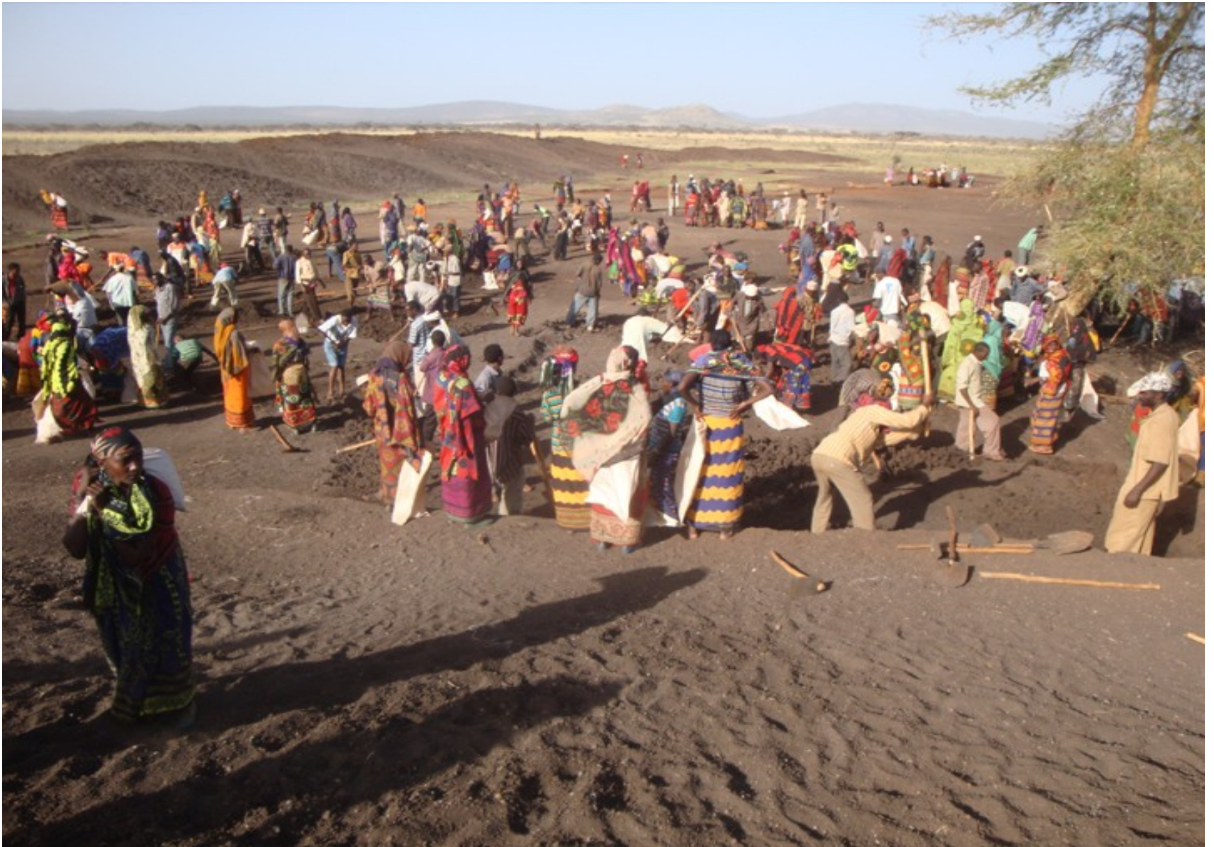
Communities excavating Melbana Pond
